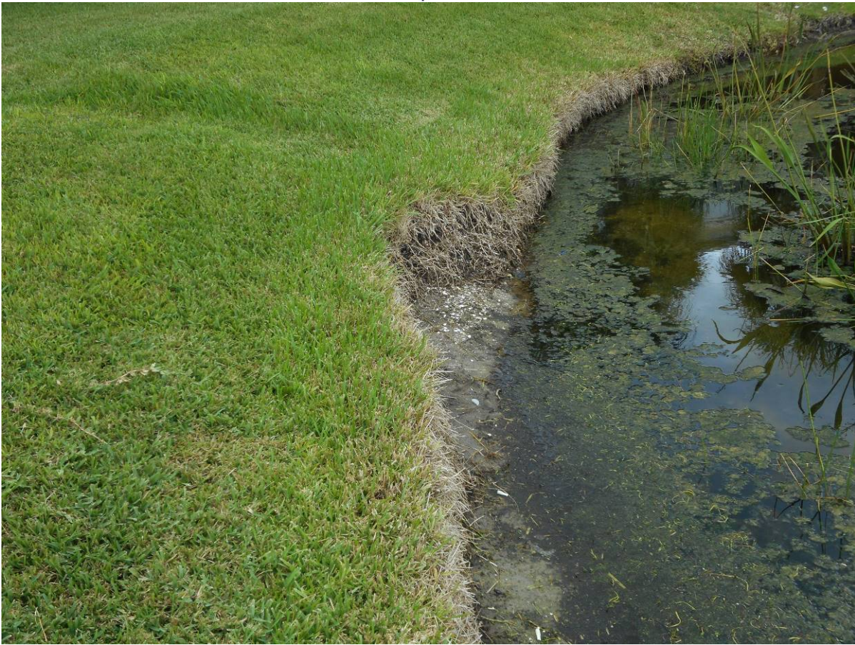
Area 1 – Minor erosion at northwest corner of Pond 5
