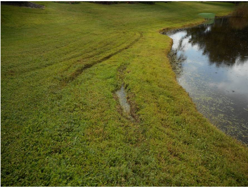
Pond 9 – South corner – erosion from mowers
