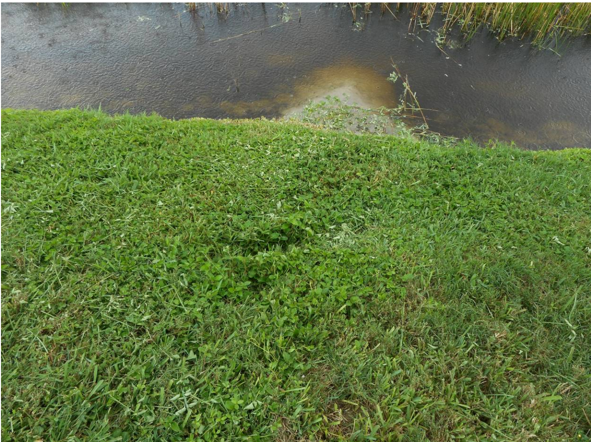
Area 4 – Minor Erosion on southwest side of Pond 8
