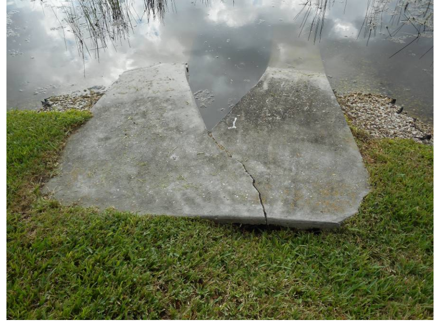
Pond 4 – East side – Cracked Mitered End Section
