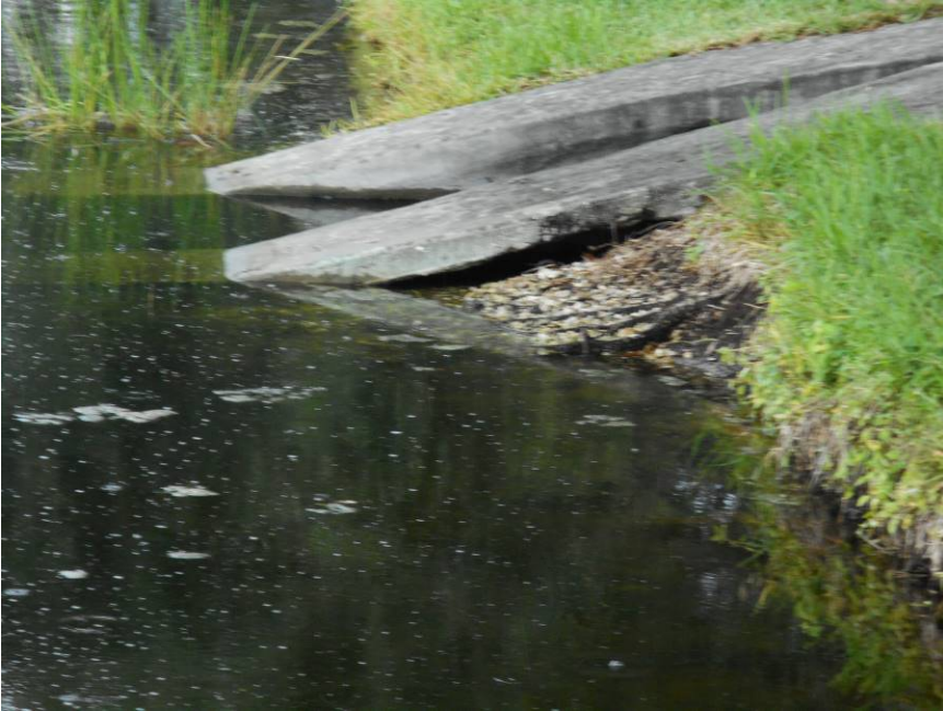
Pond 1 – Southeast corner – minor erosion at mitered end section
