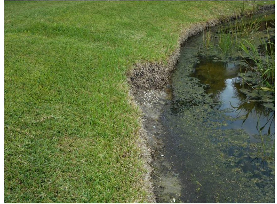
Pond 5 – Southwest corner – Minor erosion, bid package prepared
