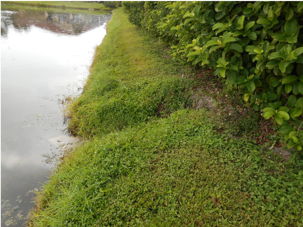
Area 3 – Erosion on west side of Pond 1
