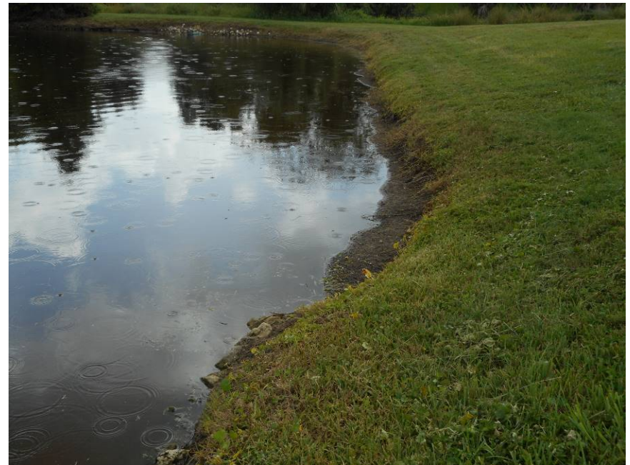
Pond 7 – Southwest side – approximately 18" of erosion
