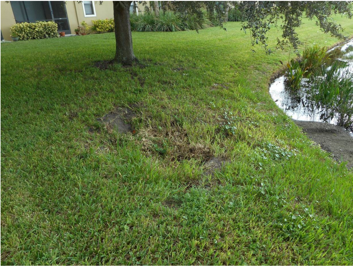
Area 2 – Approximately 6' x 8' depression at southeast corner Pond 5
