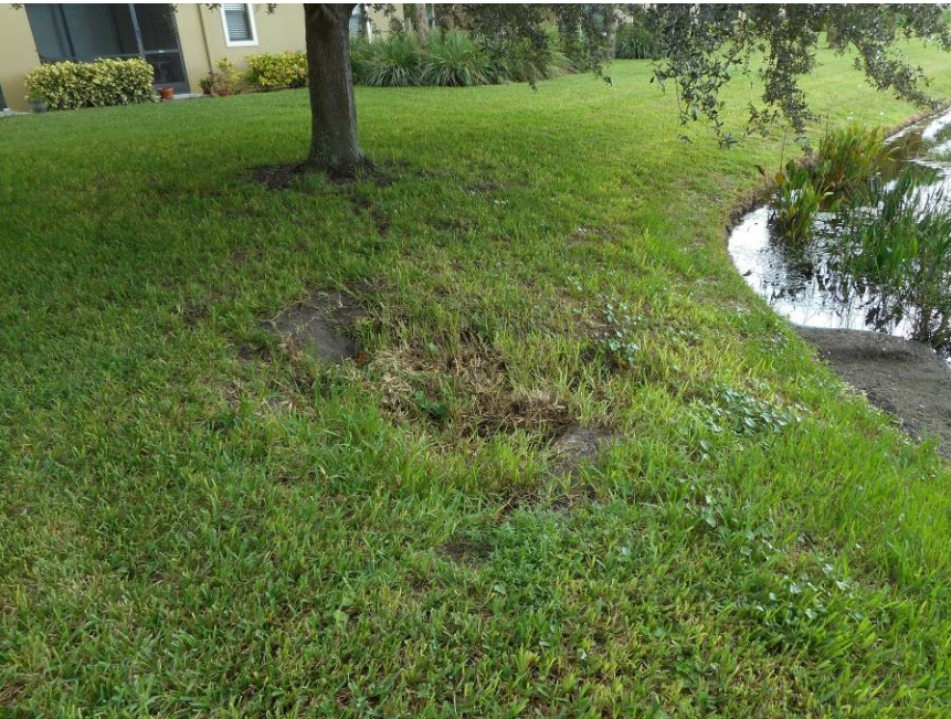
Pond 5 – Northeast corner – 6' x 8' eroded area, bid package prepared
